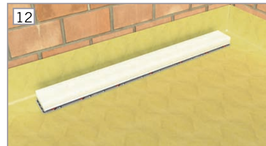
12 Protect the frame during the tiling process using the supplied cover.
