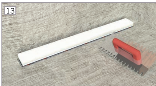
13 Fill the floor with a 1-2% slope towards the channel. Tile the walls and the floor.
